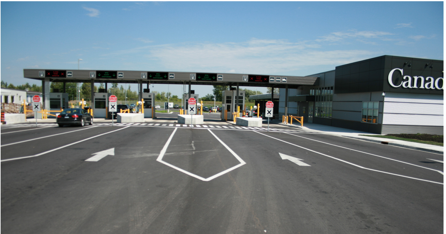
Cornwall Port of Entry, Cornwall, Ontario
